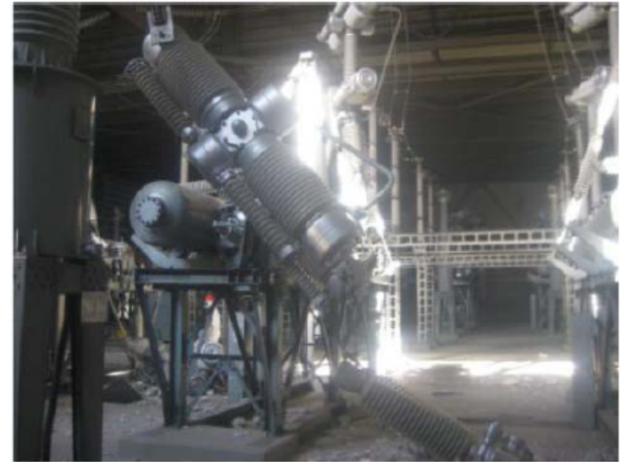
Circuit Breaker damaged
