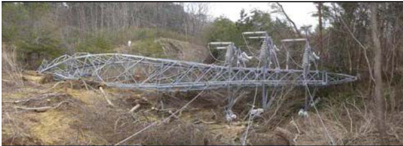
Collapsed tower
